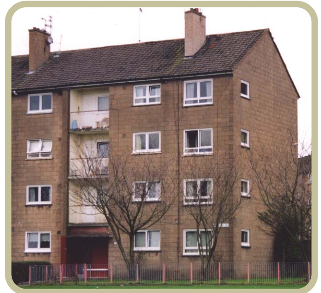
Figure 4: Typical Scottish housing of the late 1950s
