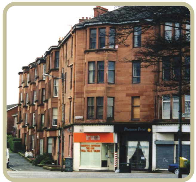
Figure 1: A typical pre-1919 red sandstone tenement
